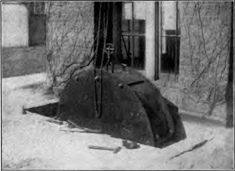
FIG. 67.—THE CASING IN POSITION.
